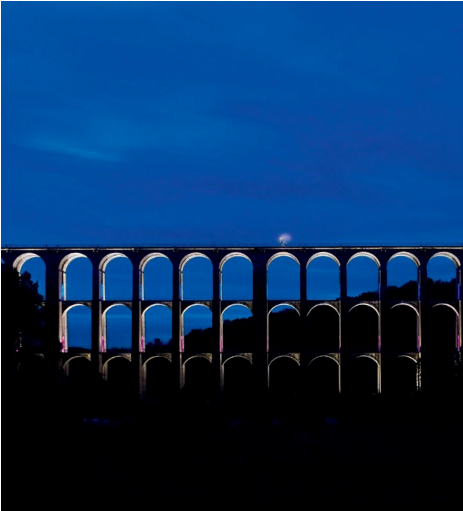
Viaduct - Chaumont, France. Architectural project: Jean Francois Touchard.
